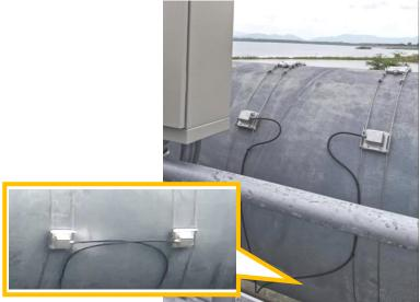
The UFL-30 series stationary, clamp-on ultrasonic flowmeter with multi-path measurement capability incorporating up to 4 pairs of transducers placed on the outside of pipes provides stable instantaneous flow rate measurements.
