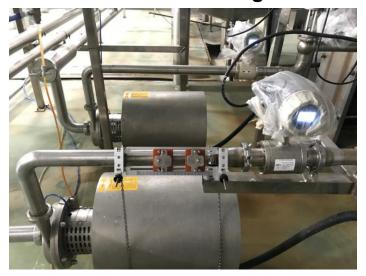
The UFP-20 portable, clamp-on ultrasonic flowmeter provides instantaneous flow rate measurements with up to 2 pairs of transducers placed on the outside of pipes.
