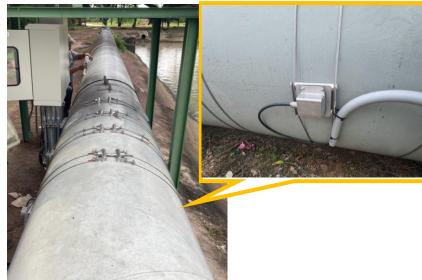
The UFL-30 series stationary, clamp-on ultrasonic flowmeter with multi-path measurement capability incorporating up to 4 pairs of transducers placed on the outside of pipes provides stable instantaneous flow rate measurements.
