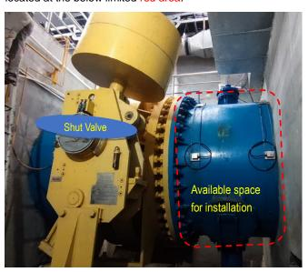
The clamp-on type ultrasonic is the best solution to be installed without stopping water or cutting pipe.
