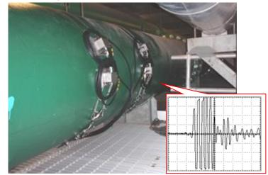
By employing the UFL-30 series stationary clamp-on ultrasonic flowmeter in combination with the appropriate sensor from the variety available and/or the system's multi-path measurement capability. You may be able to obtain high stable flow measurements of pipes from 25mm up to 6000mm in nominal diameter under less than ideal conditions.
