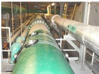
The UFL-30 series stationary, clamp-on ultrasonic flowmeter with multi-path measurement capability incorporating up to 4 pairs of transducers placed on the outside of pipes provides stable instantaneous flow rate measurements.
