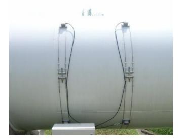
By employing the UFL-30 series stationary clamp-on ultrasonic flowmeter in combination with the appropriate sensor from the variety available and/or the system's multi-path measurement capability. You may be able to obtain high stable flow measurements of pipes from 25mm up to 6000mm in nominal diameter under less than ideal conditions.
