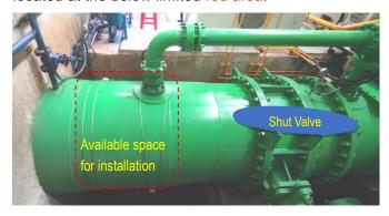
The clamp-on type ultrasonic is the best solution to be installed without stopping water or cutting pipe. Only approx. half size of pipe diameter will be required to install transducers.
