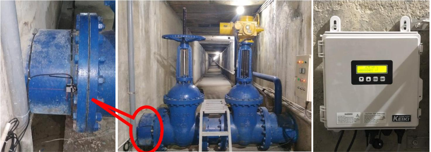
The “Intelligent digital UFW-100” stationary, clamp-on ultrasonic flowmeter with transducers placed on the outside of pipes provides stable instantaneous flow rate measurements.
