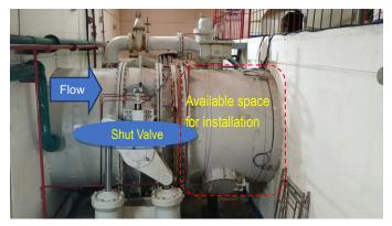
The clamp-on type ultrasonic is the best solution to be installed without stopping water or cutting pipe. Only approx. half size of pipe diameter will be required to install transducers.
