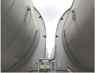
UFL can provide data of instantaneous flow rate which averaged by each diametrical axis.
