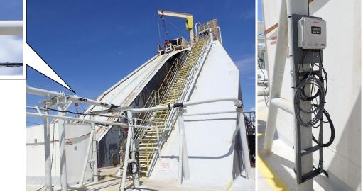
The "Intelligent digital UFW-100" stationary, clamp-on ultrasonic flowmeter with transducers placed on the outside of pipes provides stable instantaneous flow rate measurements.
