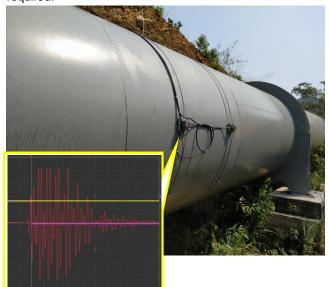
The clamp-on type ultrasonic is the best solution to be installed without stopping water or cutting pipe. Only approx. half size of pipe diameter will be required to install transducers.
