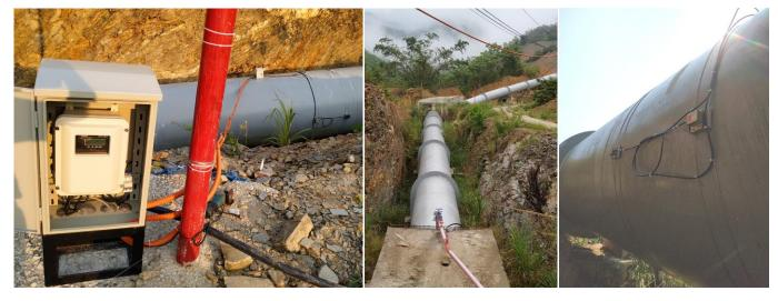
The UFL-30 stationary, clamp-on ultrasonic flowmeter with multi-path measurement capability incorporating up to 4 pairs of transducers placed on the outside of pipes provides stable instantaneous flow rate measurements.
