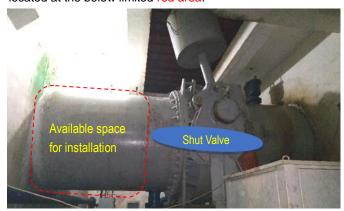
The clamp-on type ultrasonic is the best solution to be installed without stopping water or cutting pipe.
