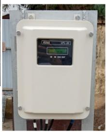
The UFL-30 series stationary, clamp-on ultrasonic flowmeter with multi-path measurement capability incorporating up to 4 pairs of transducers placed on the outside of pipes provides stable instantaneous flow rate measurements.
