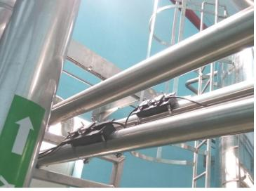
The "Intelligent digital UFW-100" stationary, clamp-on ultrasonic flowmeter with transducers placed on the outside of pipes provides stable instantaneous flow rate measurements.
