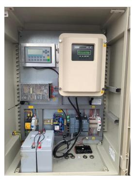
The UFL-30 series stationary, clamp-on ultrasonic flowmeter with multi-path measurement capability incorporating up to 4 pairs of transducers placed on the outside of pipes provides stable instantaneous flow rate measurements.
