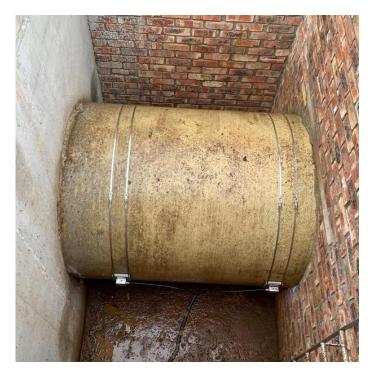
The UFL-30 series stationary, clamp-on ultrasonic flowmeter with multi-path measurement capability incorporating up to 4 pairs of transducers placed on the outside of pipes provides stable instantaneous flow rate measurements.
