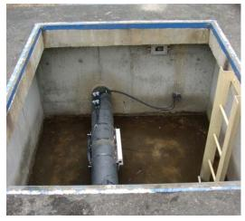
The "Intelligent digital UFW-100" stationary, clamp-on ultrasonic flowmeter with transducers placed on the outside of pipes provides stable instantaneous flow rate measurements.
