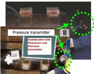
The UFL series stationary, clamp-on ultrasonic flowmeter with multi-path measurement capability incorporating up to 4 pairs of transducers placed on the outside of pipes provides stable instantaneous flow rate measurements.
