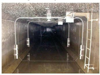
The UF960 series stationary, clamp-on ultrasonic flowmeter with multi-path measurement capability incorporating up to 2 pairs of transducers placed inside channel provides stable instantaneous flow rate measurements.
