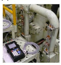
The UFP-20 portable, clamp-on ultrasonic flowmeter provides instantaneous flow rate measurements with up to 2 pairs of transducers placed on the outside of pipes.
