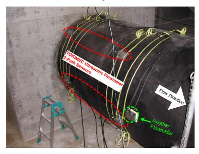
The UFL-20 series stationary, clamp-on ultrasonic flowmeter with multi-path measurement capability incorporating up to 4 pairs of transducers placed on the outside of pipes provides stable instantaneous flow rate measurements.
