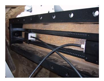
Although such buried or underground installations should normally be avoided for reasons of maintenance, conditions may dictate this mode of installation. In such cases a multi-path installation enables a higher degree of stability in measurement providing a viable long term, low-maintenance alternative.
