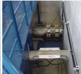
The UFL-20 series stationary, clamp-on ultrasonic flowmeter with multi-path measurement capability incorporating up to 4 pairs of transducers placed on the outside of pipes provides stable instantaneous flow rate measurements.
