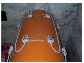
Although a 50-fold (or "50D") pipe diameter length of straight run downstream from the pump outlet is normally required for proper measurement, stable measurements-even in applications such as this where straight run lengths are insufficient - can be achieved by applying multi-path measurement methods.
