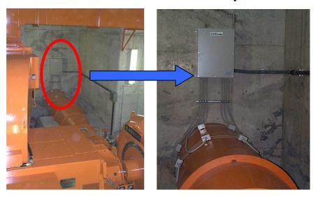
The UFL-20 series stationary, clamp-on ultrasonic flowmeter with multi-path measurement capability incorporating up to 4 pairs of transducers placed on the outside of pipes provides stable instantaneous flow rate measurements.
