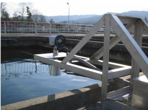
The MRG-10 micropower impulse radar level gauge features accurate, non-contact, level measurement with simple installation over a target fluid.
