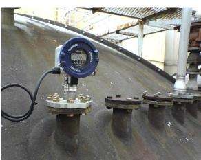
The MRG-10 micropower impulse radar level gauge features accurate, non-contact, level measurement with simple installation over a target fluid.
