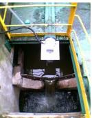
The MRG-10 micropower impulse radar level gauge features accurate, non-contact, level measurement with simple installation over a target fluid.
