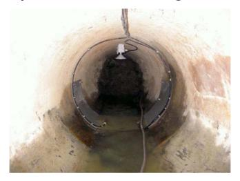
The UVH-2000 series stationary, clamp-on ultrasonic flowmeter with multi-path measurement capability incorporating up to 2pcs of transducers placed inside channel provides stable instantaneous flow rate measurements.
