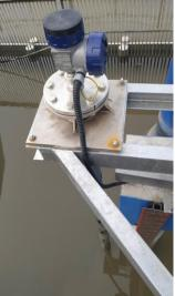
The KRG-10 micropower impulse radar level gauge features accurate, non-contact, level measurement with simple installation over a target fluid, in this case, river waters.
