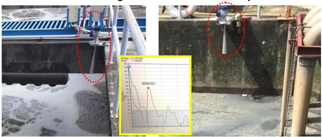
The KRG-10 micropower impulse radar level gauge features accurate, non-contact, level measurement with simple installation over a target fluid.
