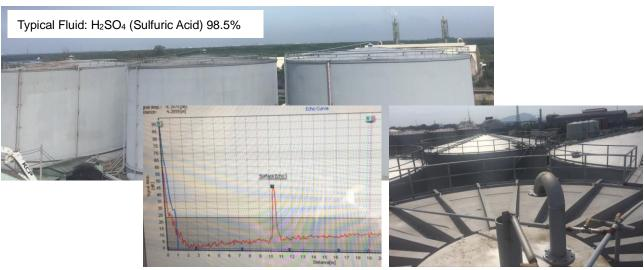
The KRG-10 radar level gauge features accurate, non-contact, level measurement with simple installation over a target fluid. In applications such as acid process liquid tanks where the sensing elements of contact type level instruments are exposed to corrosion and substance adhesion, non-contact means of measurement which are unencumbered by such concerns are preferable for durability and reliability of measurement.
