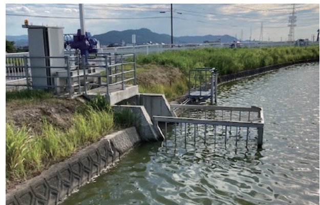
Reservoir gate automation equipment
