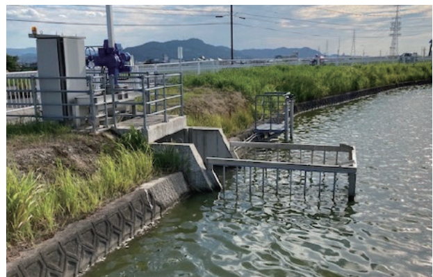
Reservoir gate automation equipment
