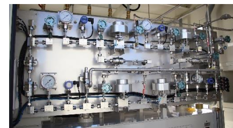
Hydrogen compression equipment in the Fukushima Hydrogen Refueling Technology Research Center
