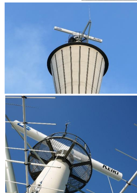
The radar installed atop an approx. 110-meter tall tower
