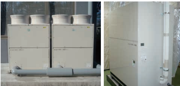
Sequential replacement of water-cooled air conditioners with energy-saving air-cooled models
